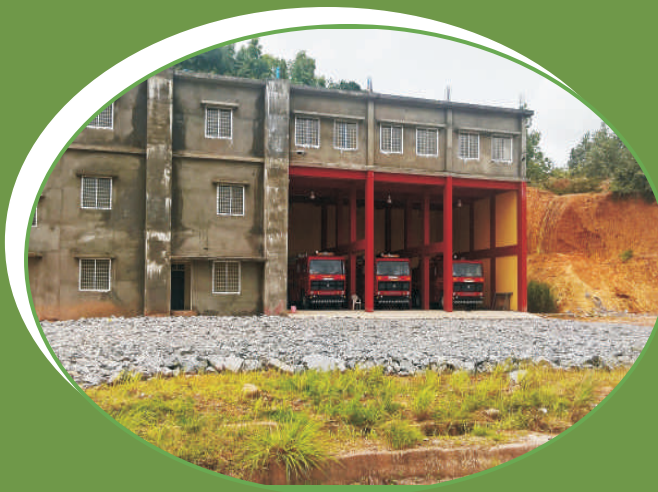
24/7 Fire Tenders in operation
